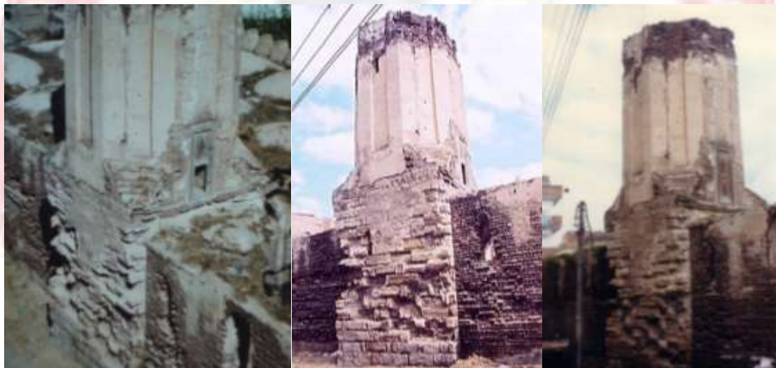
Pl. 9. Three pictures of the western minaret, which shows the rinsing of inverted triangles to convert the square section of the base of the minaret to the octagon, as well as the octagonal floor built with carved bricks and the square base built with stone
