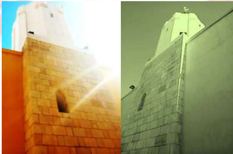
Pl. 6. Two pictures of the minaret after faulty restoration and alteration of monuments by canceling the transition area between the square and octagonal sectors
