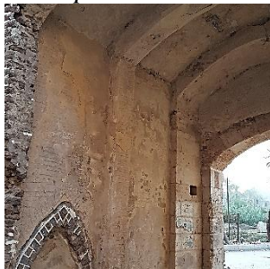
pl. 3. Details of the vault mounted on arches and the vaulted niche to sit the guard on the right side of the gate
