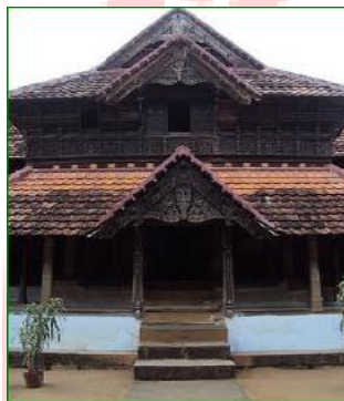
Figure 5: Roof of Padmanabhapuram palace, Kerala- a palace done in the vernacular style for the erstwhile ruling family of Kerala.
