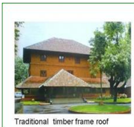
Figure 18: Traditional timber frame roof. Source: Pillai, H. (2004) in http://www.archiestudio.in/ . (Accessed in July 2016)
