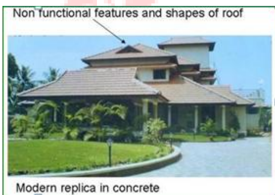
Figure 19: Modern Day interpretation of the Traditional timber frame roof in concrete in Kerala. Source: Pillai, H. (2004) in http://www.archiestudio.in/ . (Accessed in July 2016)
