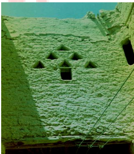
Pl. 25. Ventilation holes for houses from Unaizah
