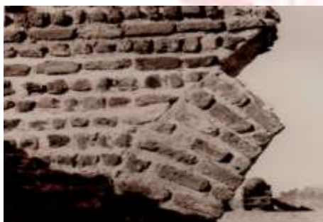
Pl. 6. The second entrance at Al-'Abed Castle
