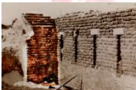
Pl. 5. Entrance lobby at Al-'Abed Castle
