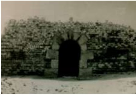
Pl. 12. The northwestern façade of Al-'Abed Castle
