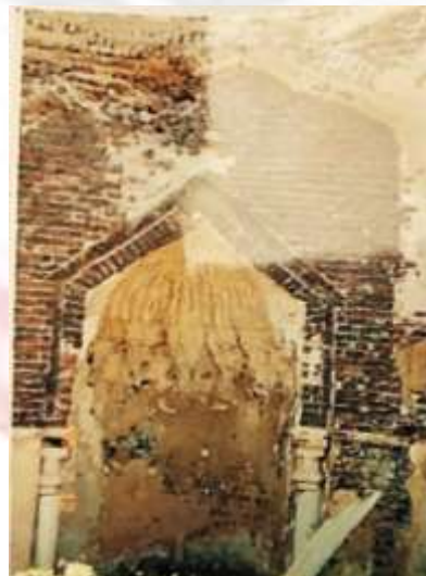
Pl. 1. The picture that was relied on for the restoration shows remnants of stucco on the faces of the bricks after the decorations have fallen off
