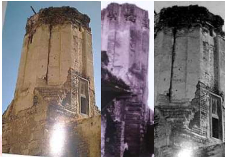
Pl. 8. Three pictures of the western minaret, which shows the rinsing of inverted triangles to convert the square sector of the minaret base to an octagon, also shown is the octagonal floor built with hinged bricks
