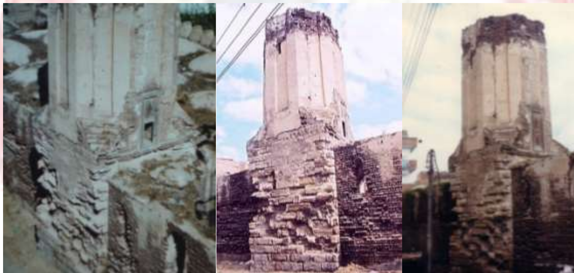
Pl. 9. Three pictures of the western minaret, which shows the rinsing of inverted triangles to convert the square section of the base of the minaret to the octagon, as well as the octagonal floor built with carved bricks and the square base built with stone
