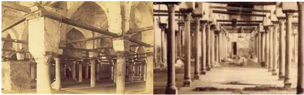
Pl. 13. The ancient columns of the mosque are of different models, which have been replaced by modern ones
