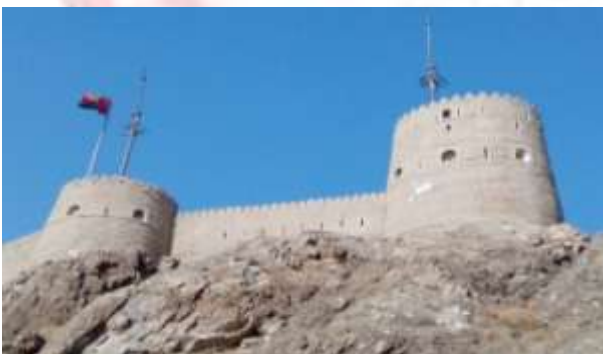
(Fig. 10) The general shape of the east and southeast towers from outside the castle (Photo by the researcher)
