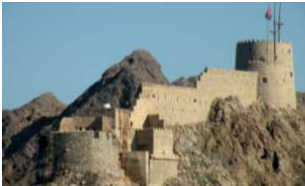
(Fig. 14) shows the exterior shape of Muttrah fort
