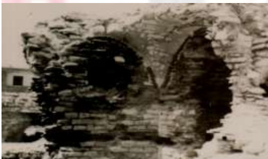
Pl. (6). The inner tower of the Rosetta Castle, from:Darwish, Mahmoud Ahmed. Encyclopedia of Rosetta, 1, plate 40.
