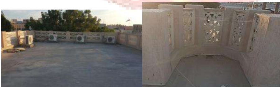
pl. 32) The roof of al-Shoyoukh Mosque (the summer prayer hall)
