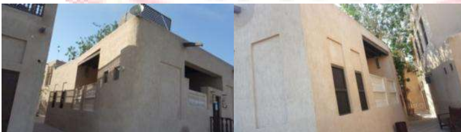
pl. 5. The northern façade of the IbnZayed Mosque
