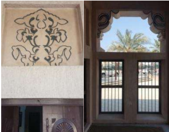
pl. 65. The north wall of the mosque portico
