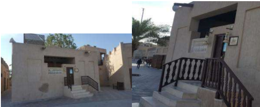
pl. 3. The m'Ain eastern façade of the Ibn Zayed Mosque
