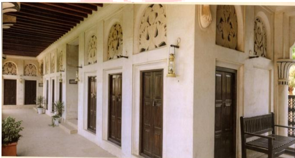
pl. 12. Plaster windows above the rooms on the upper floor
