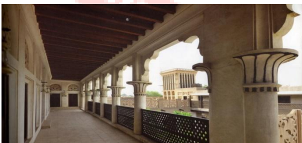
pl. 11. Upper Liwan after restoration
