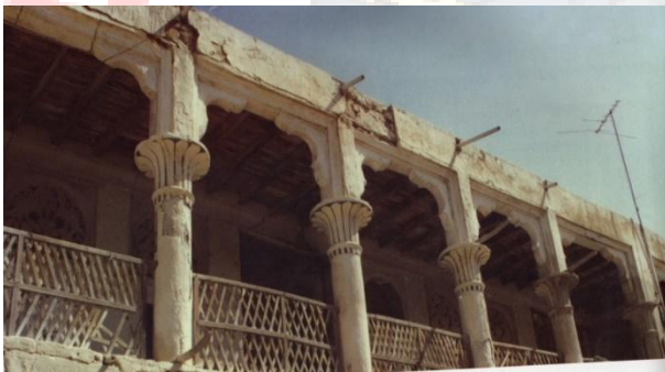
pl. 10. Upper Liwan before restoration
