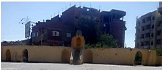
pl. (7) The pulpit and the wall of the qibla in the Eid prayer hall in Aswan on the authority of Dr. Muhammad Abdul Rahman
