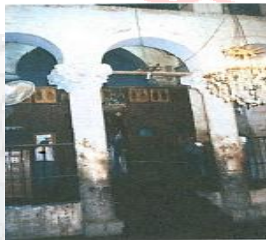
Pl. 4. Models of the semi-circular arches supporting the upper floor and the dome in the Church of the Virgin in Jabal Al-Tair
