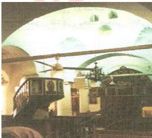
Pl. 3. the semi-circular arches supporting the dome of the nave in the monastery of al-Azab church
