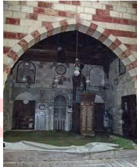
pl. 20. the Pentagonal pointed arch that decorates the facade of the entrance to the qibla iwan in Mohib al-Din al-Tayyib Mosque
