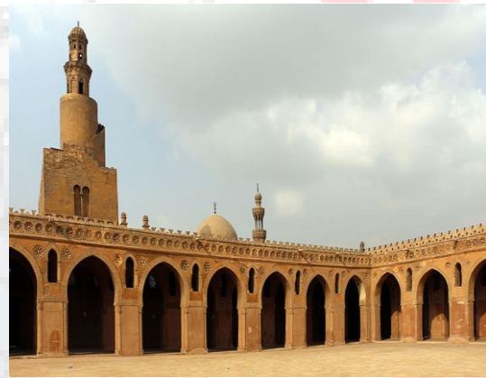
Pl. 16. models of the pointed arches with two centers in the Ahmed Ibn Tulun Mosque
