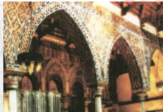
pl. 22. Models of the Pentagonal pointed arches supporting the gabled roof of the Hanging Church
