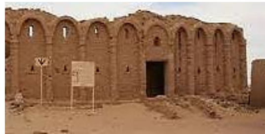
pl. 32. A group of semi-circular solid arches adorning the facade of one of the Begawat shrines
