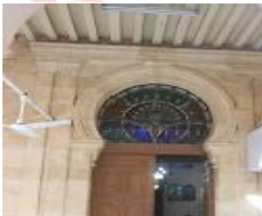
Pl. 23. A flat arch that crowns one of the entrances to the monastery of Angel Gabriel in Abdeen
